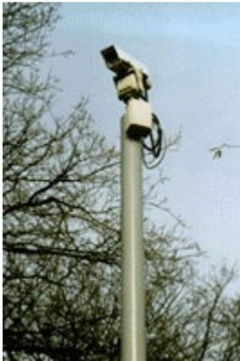
Exterior cameras should have pan, tilt, and zoom capabilities. In areas where inclement weather may obscure monitoring, they should be enclosed in secure, weather-tight boxes with heat, wash, and wipe capabilities.
