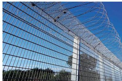
Razor wire can be installed above the barbed wire outriggers if additional security is desired. Steel posts can be set in concrete and bottom rails or tension wires can be installed at the base of the fabric. A trench at the base of the fence can be filled with concrete to prevent tunneling.
